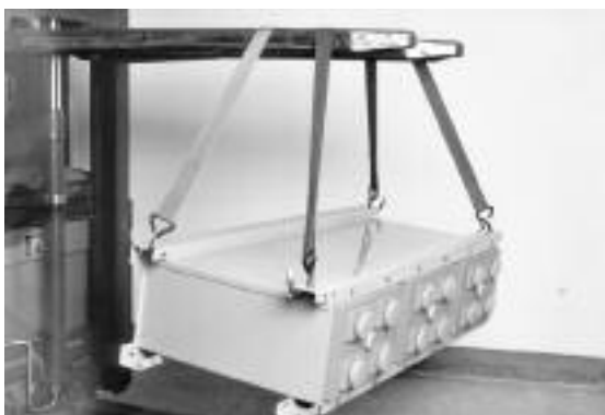
Figure 5: Positioning the module onto the base channels
