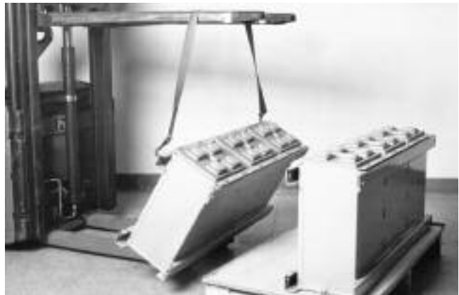
Figure 4: Lifting the module clear of the pallet
