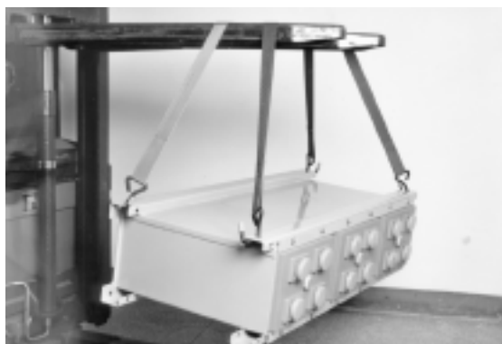
Figure 5: Positioning the module onto the base channels
